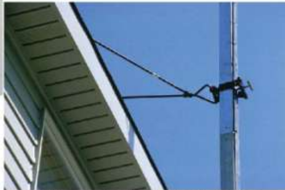
A Pump Jack scaffold's triangular bracing.
